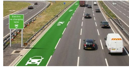
Fig. 18. Charging on the go (Inductive) [15].
